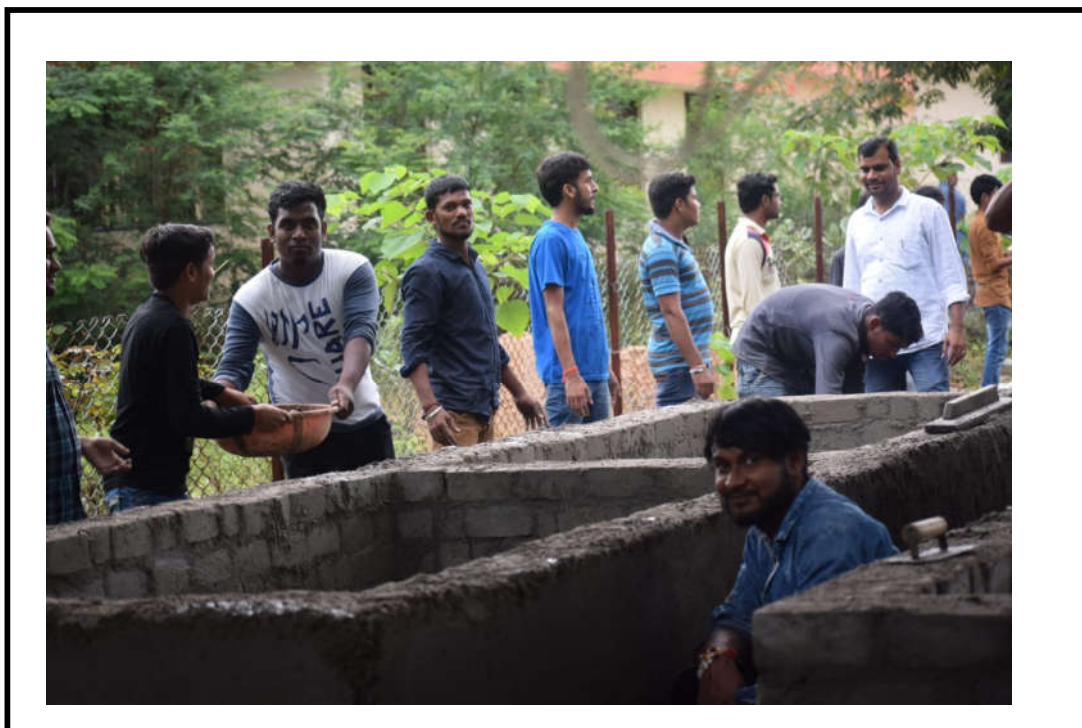
Construction of Vermicompost Unit
