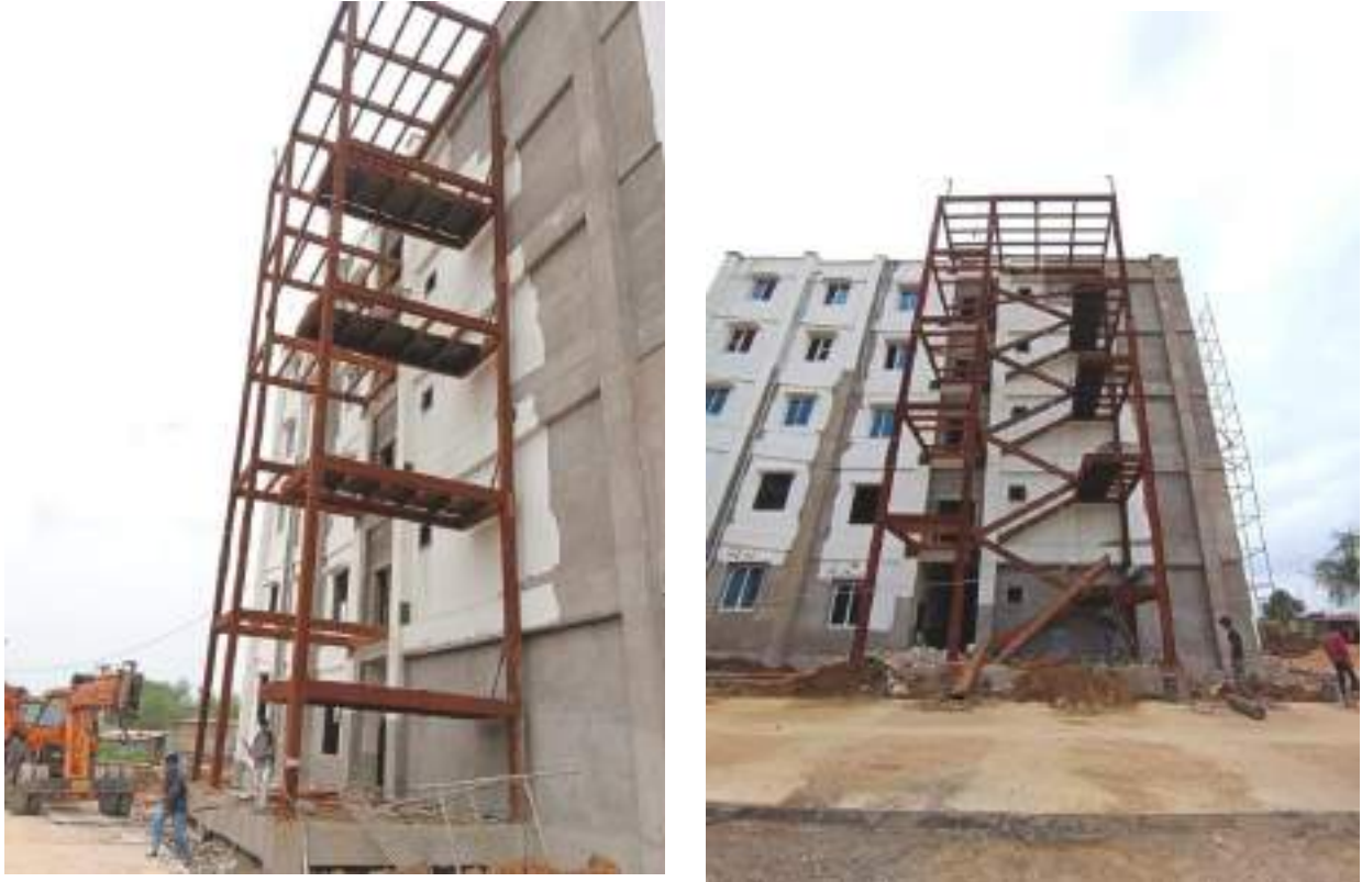
Fig 9: Fire safety provision
