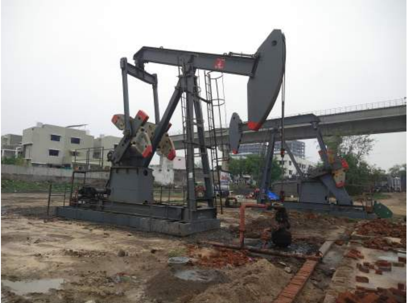
Fig. 7: Beam Pump Unit (Pumpjack)
