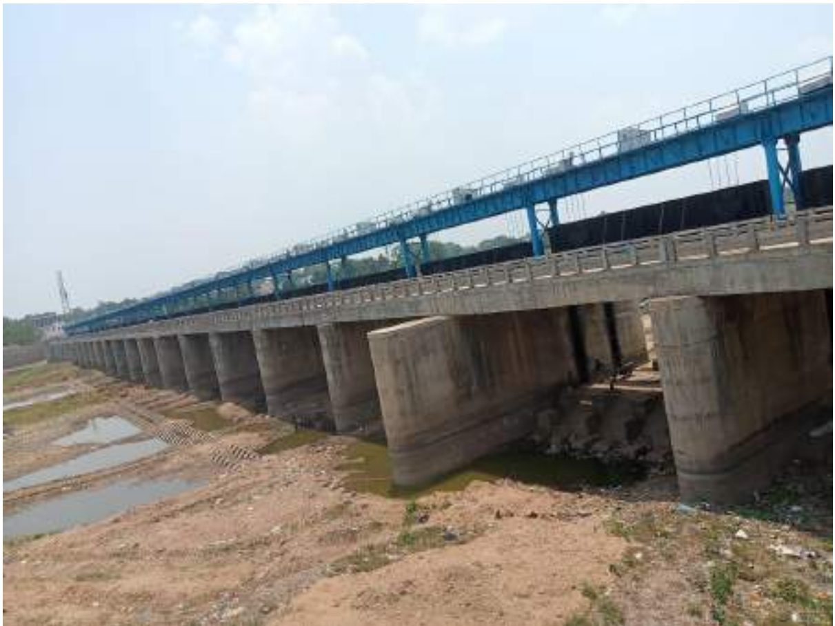
Fig. Shivghat Barrage, Arpa river, Bilaspur
