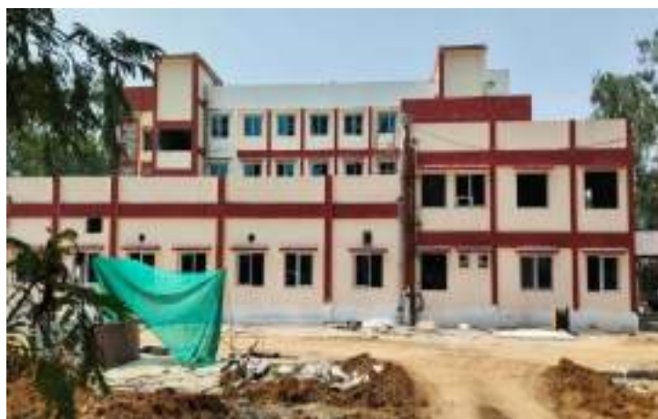
Figure 3: Side View of Girls Hostel (250 seats) Under Finishing
