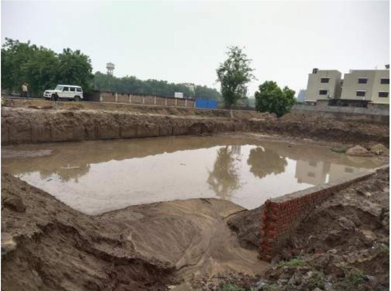
Fig. 6: Cutting Pit Under Construction.
